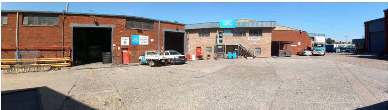
Photo 3 - General Site Conditions - North part of the site looking South
